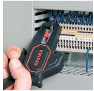
Stripping in confined areas
